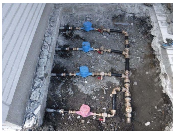
[鉛製給水管更新の様子]
