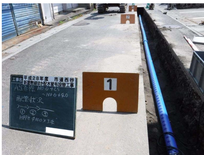
[配水管布設替の様子]
